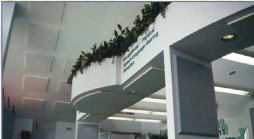
Sound Delete Acoustical Ceiling Panels and Wall Panels to reduce noise reflection of drywall ceiling
