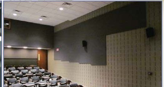
Sound Delete Acoustical Wall Panels on wall to reduce noise reflection
