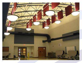
Many ceilings in recreational facilities provide virtually no acoustical contribution. Exposed bar joists and metal deck, gypsum board, preformed concrete and wood are the most common. Flush mounting acoustical panels (actually wall panels applied to the ceiling) work well and can be sized and patterned to avoid lighting, air conditioning vents, sprinklers or other obstructions.
